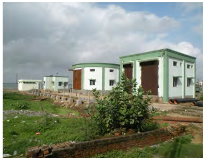
Fig. 7 : Sewage treatment plant near Bichhia nallah, Kuraghat, Gorakhpur.
